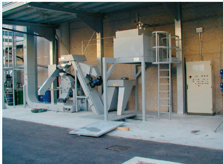
Detail of the spun swarf discharge area
