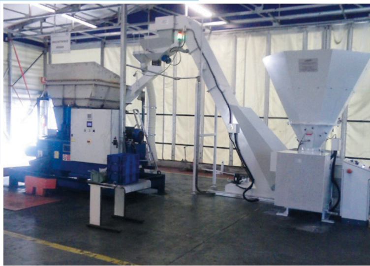
Automatic crushing and briquetting system
